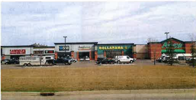
Existing commercial uses adjacent to Highway 27.
