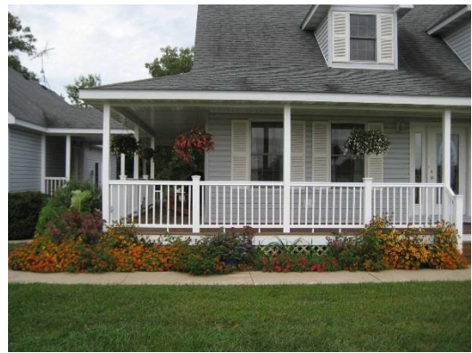
Covered front porch treatment
