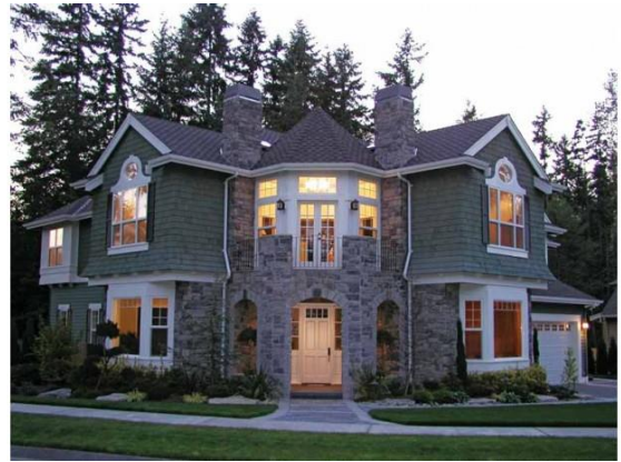
Corner unit with similar level of architectural detailing as the front elevation
