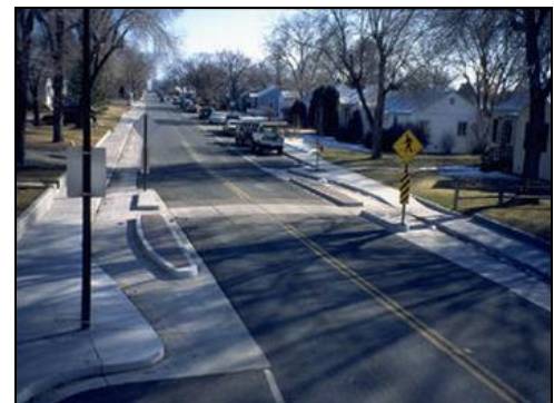
Bulb outs and curb cuts.
