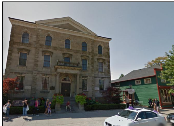
Exterior of older building is maintained while interior is renovated to accommodate new use.
