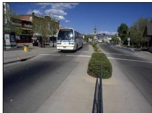
Raised medians with plantings.
